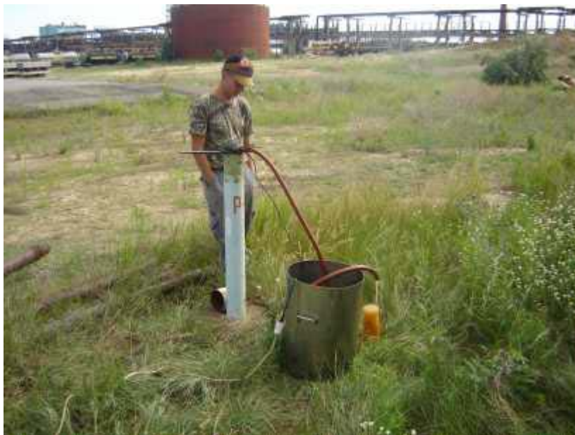
Fig. 2. Groundwater pumping out of an observation borehole
